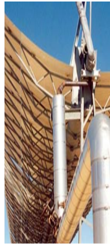
Concentrated Solar Power
